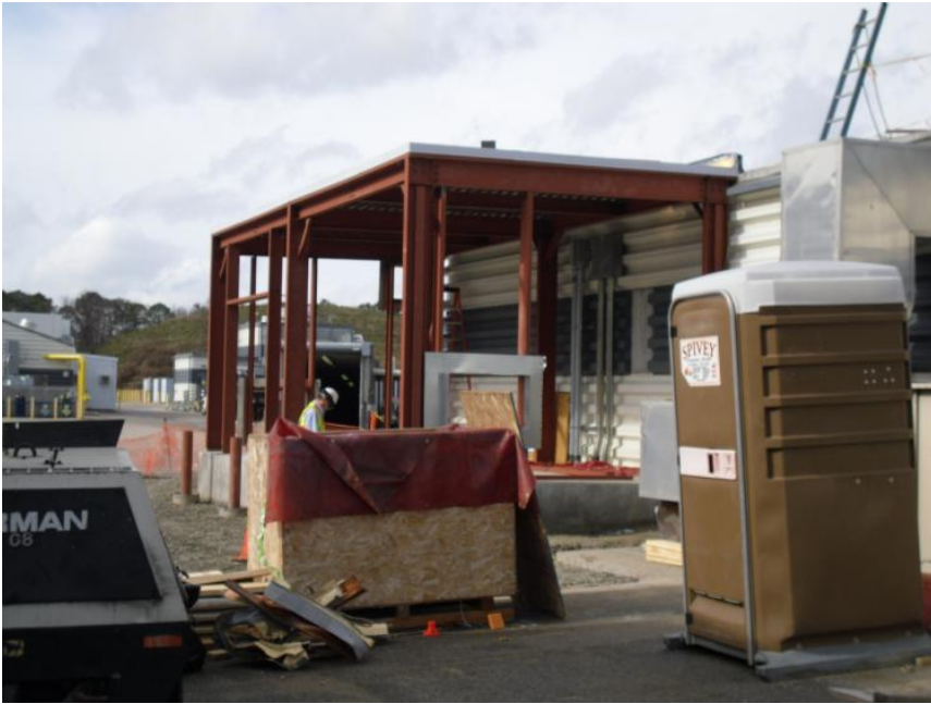
B68 (W2) addition
