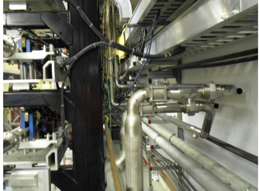
B68 tunnel LCW modifications
